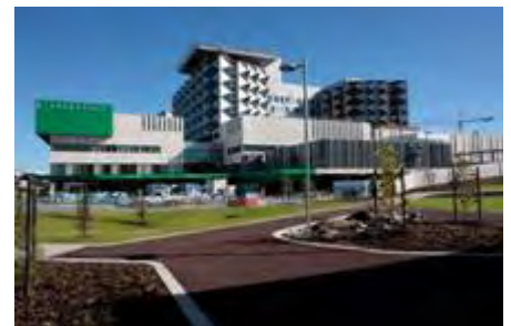
Fiona Stanley Hospital
